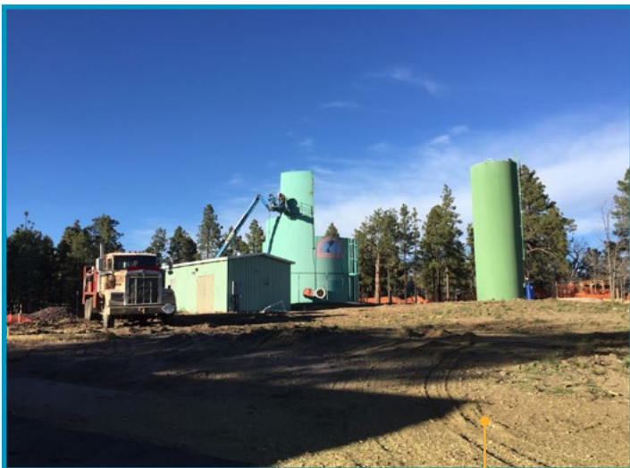
Removal of the old water tanks | Image: Dyer Lytle
