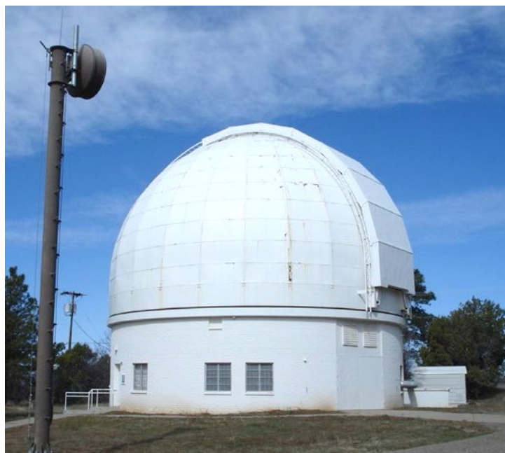
Image: The Perkins 72-inch Telescope enclosure at Anderson Mesa. In the foreground, the microwave mast and antenna which provides high-speed data communications with Mars Hill.
