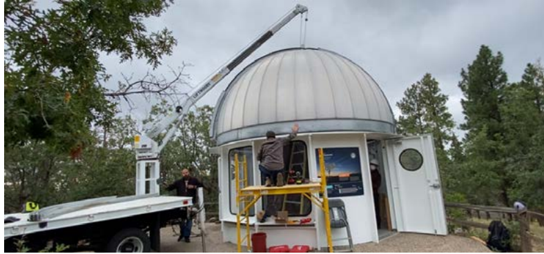
Re-installing the rails on the Dyer Telescope dome.
