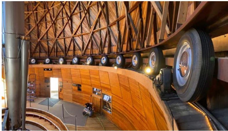
The new and improved tires on which the Clark Telescope dome rotates.
