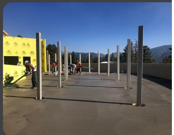
View of the Skylight Terrace looking north as the concrete slab is poured.
